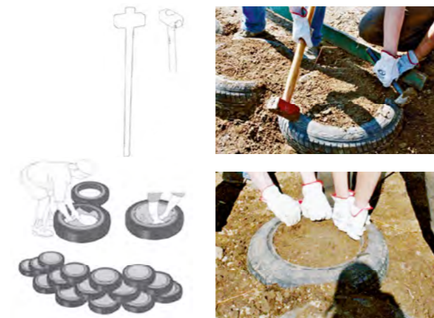
Tyres filling: It's important to fill completely the tyres. First with hands press the soil, then use the hammer to obtain a very compact soil.
