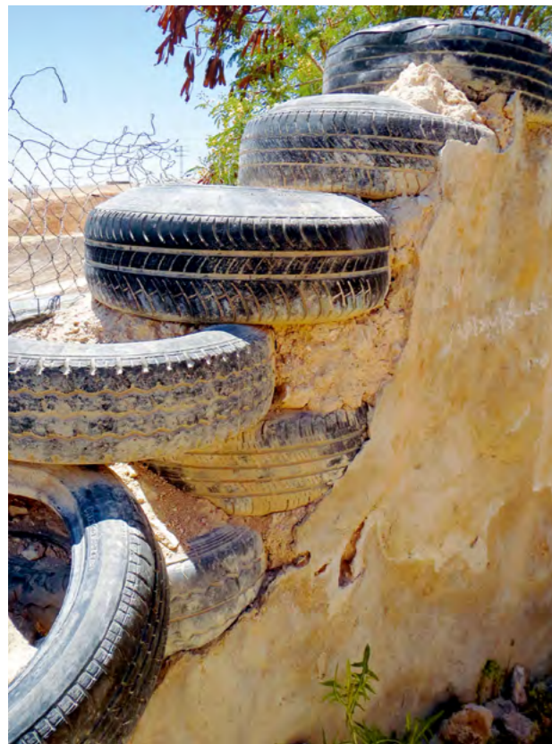
Tyres filling: It's important to fill completely the tyres. First with hands press the soil, then use the hammer to obtain a very compact soil.
