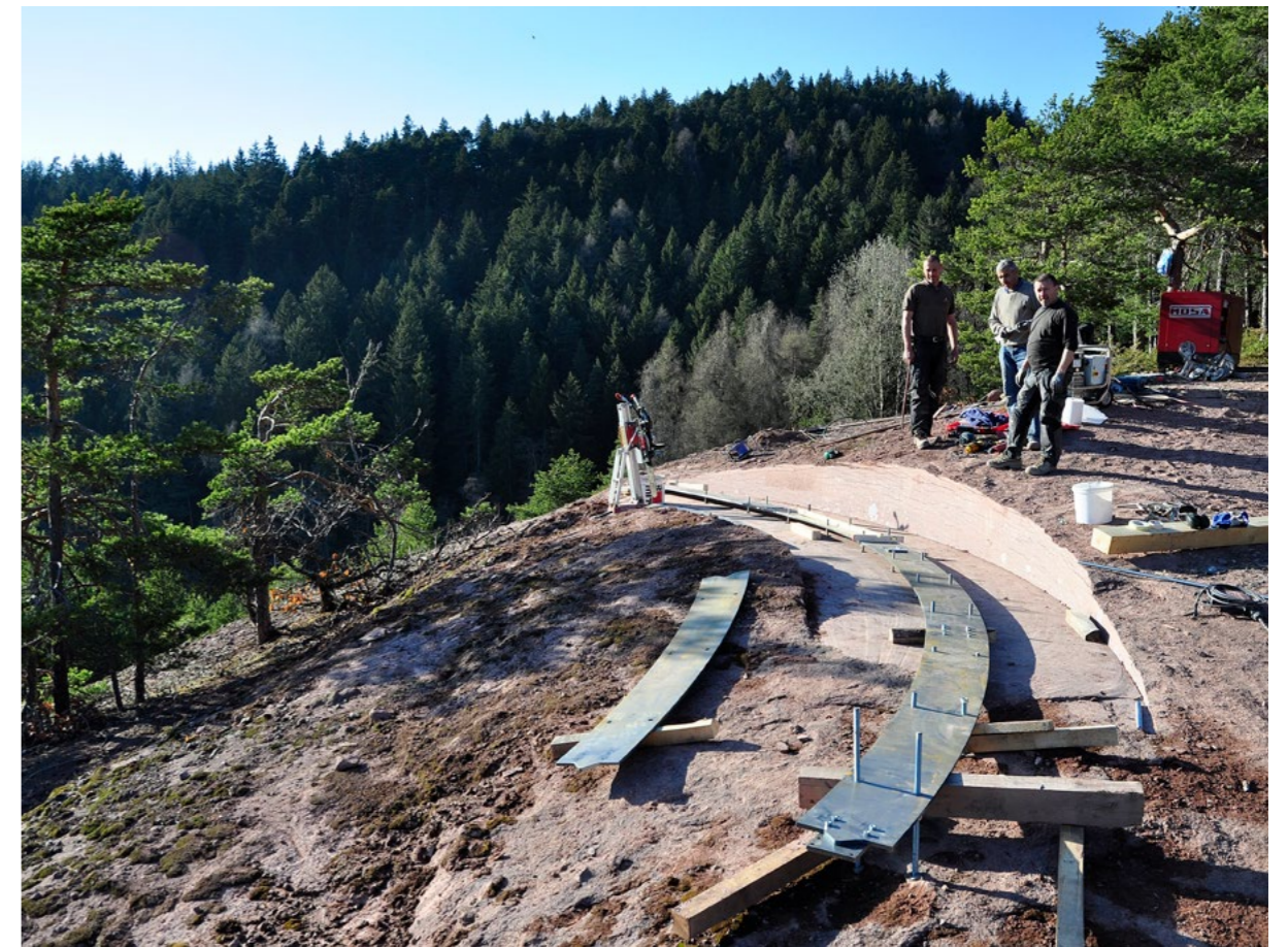
Timpfler-Knott Construction site Photo Messner Architects
