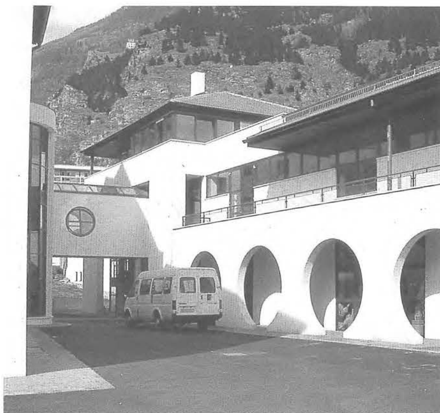
Behindertenheim Schlanders/Centro per disabili a Silandro, (W. Gadner)
